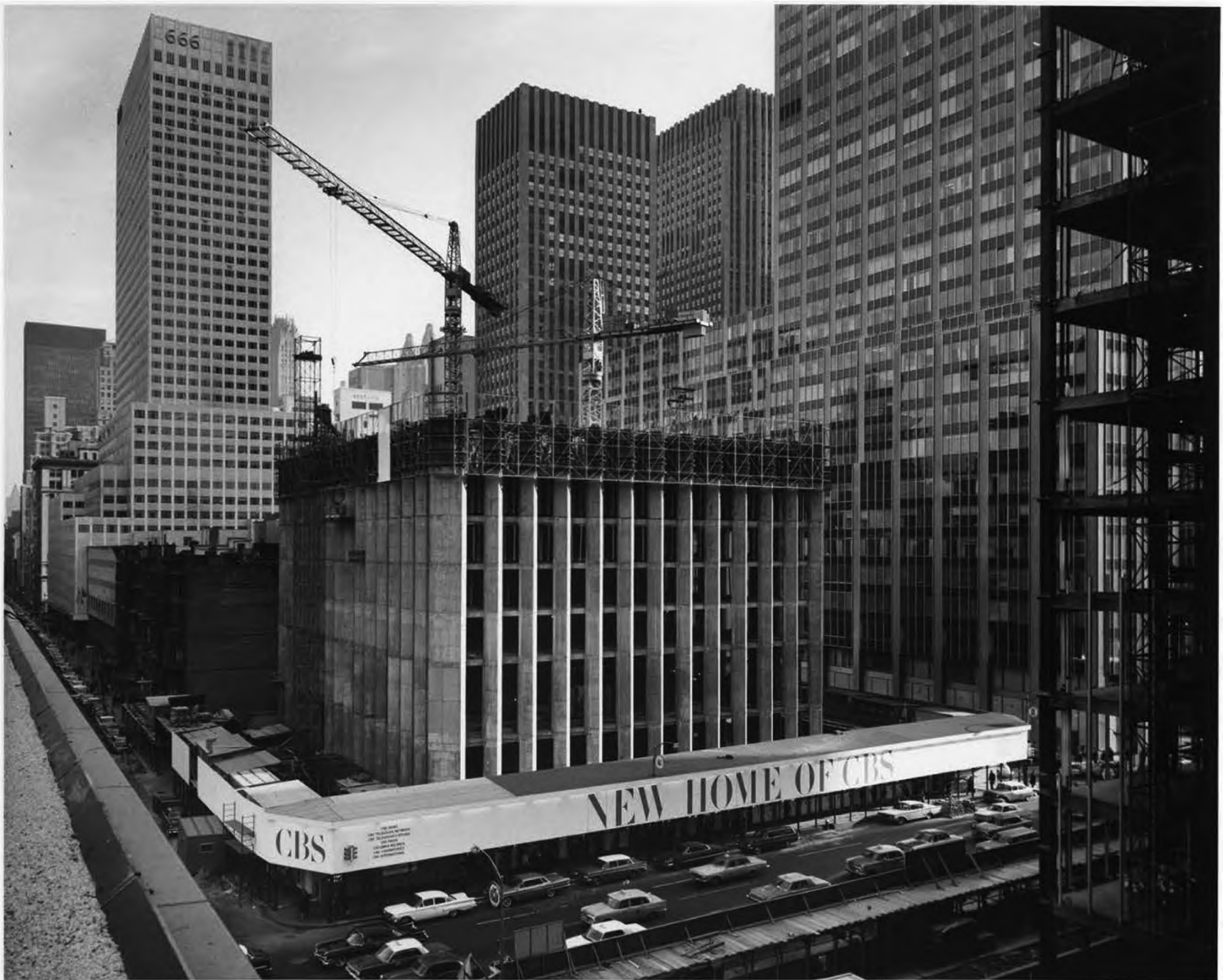
Figure 5. CBS building under construction, New York, 1965. Architect, Saarinen; Engineer, Paul Weidlinger. (Saarinen Collection, Manuscripts and Archives, Yale University.)
