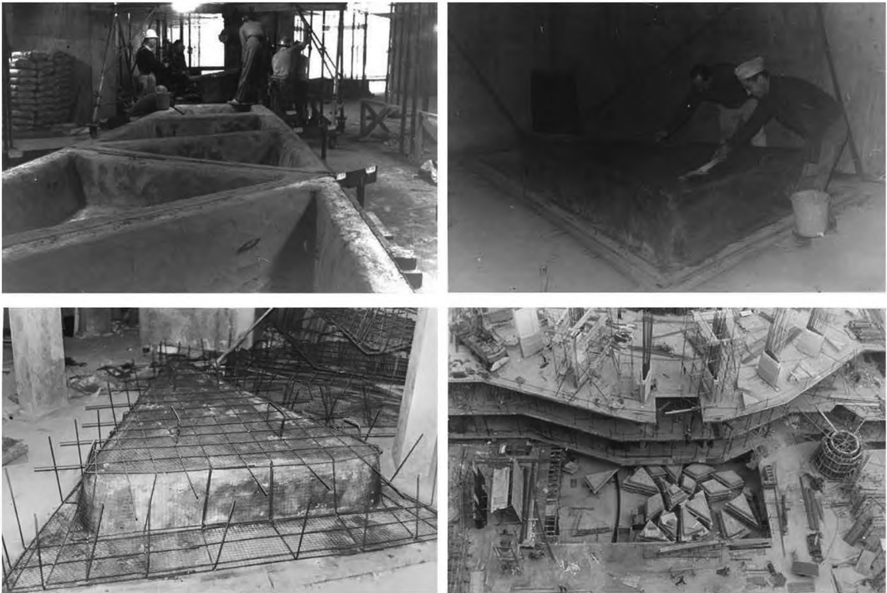
Figure 15. Top left: rendered bricks master mould; Top right: preparation of secondary mould; Bottom left: ferro-cemento panel; Bottom right: ferro-cemento panels; Sydney, 1965. (Lend Lease Historical Archive.)
