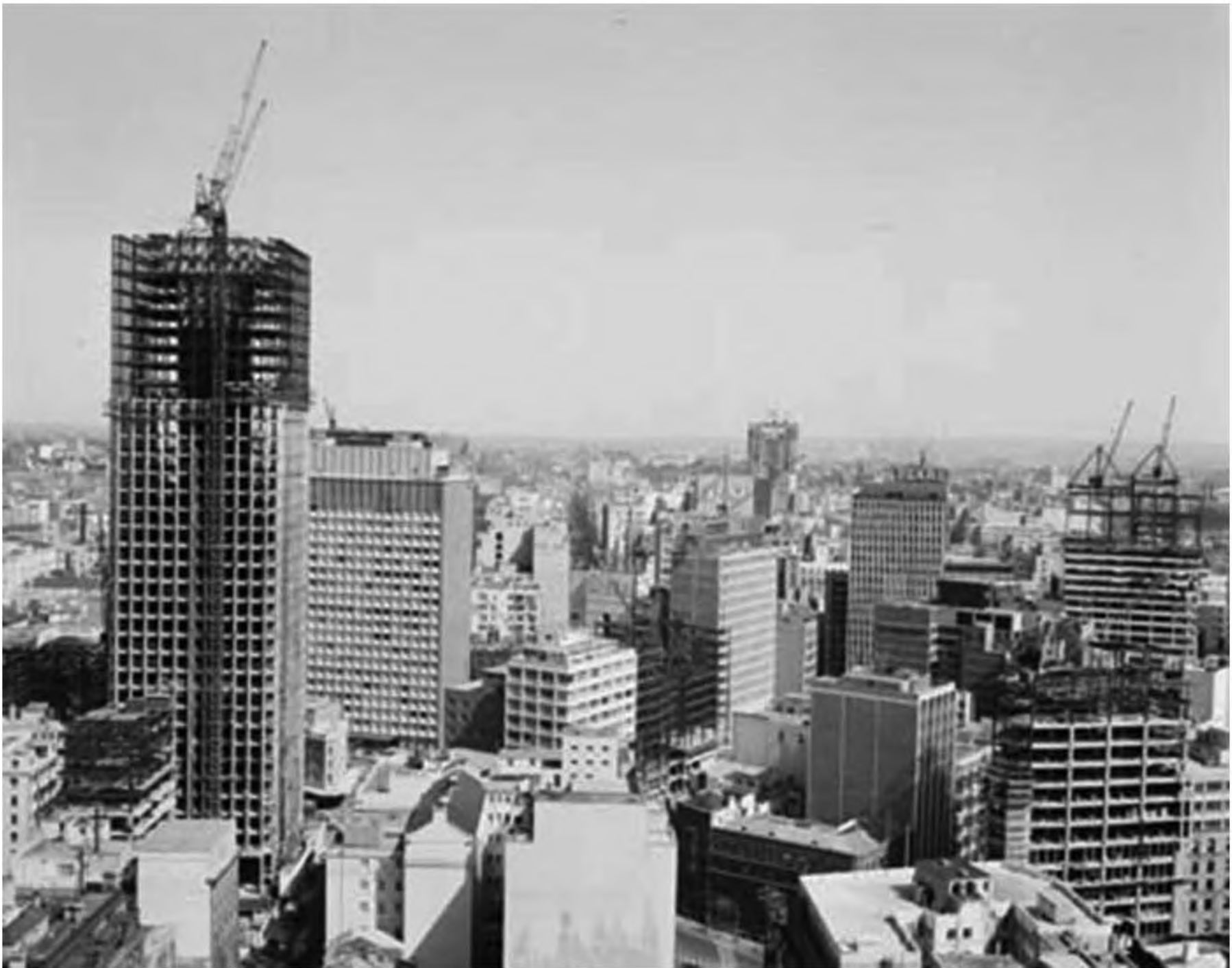
Figure 3. Changing Sydney skyline, 1964. On the left side the State Office Block under construction. Architect, Ken Woolley; Engineer, TTW Pty Ltd. (City of Sydney Archives). (Photo: A. Ozolins. National Archives of Australia.)
